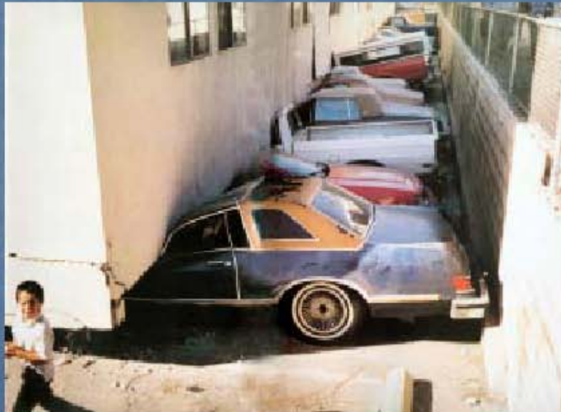
Apartment building with first storey collapse
