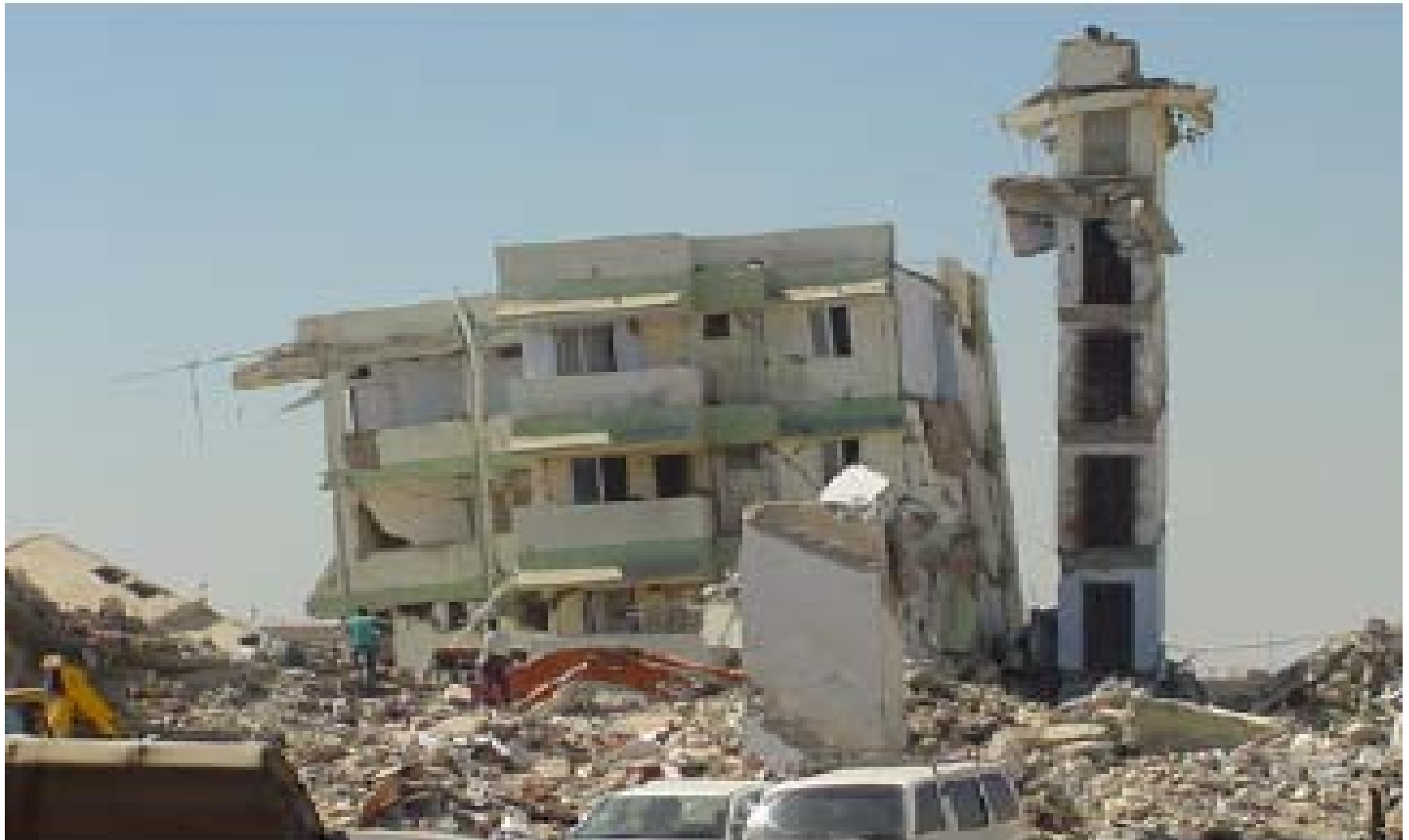
Figure 10-65. Improper anchorage into stiff RC elevator core walls in Gandhidham.
