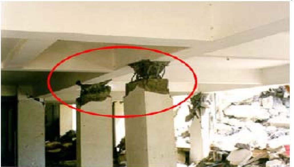
Figure 10-24. Failure of the weak concrete in the topi just below the beam (Bhuj).
