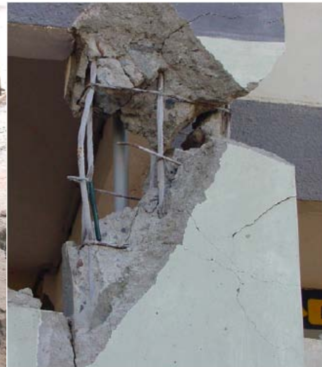
Figure 10-34. Shear failure.
