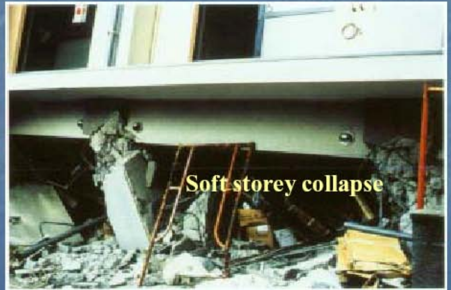
First storey collapse residential building
