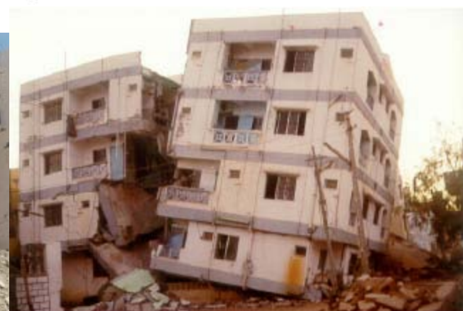
Figure 10-40. Collapse of a partially open ground story building in Bhuj, coupled with vertical split of the building at the midline.
