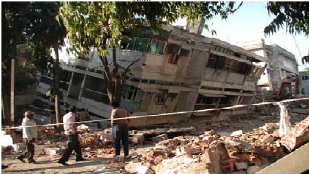
Figure 10-29. Complete collapse of apartment
